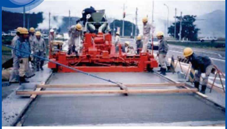
A thin layer of concrete is laid on top of the existing, deteriorated concrete pavement to restore its surface properties.
